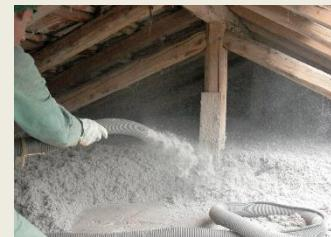
Fig 2: Cellulose insulation in open attics
