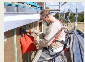
Fig 4: Cellulose insulation in a wall
