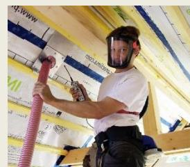
Fig 3: Cellulose insulation in a pitched roof
